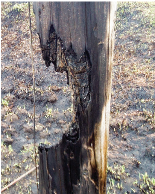
Before burning, check the property for electrical equipment and power poles to avoid damage and potential outages.
